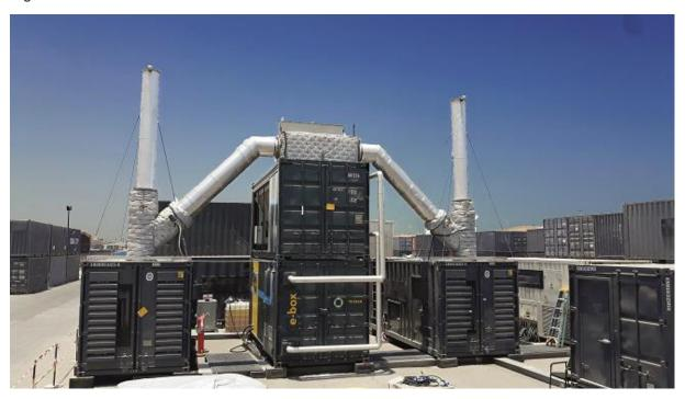
The Dutch manufacturer Triogen has developed a containerized "e-box", a solution that is tailor-made for remote mine sites. It has been designed for easily upgrading any diesel genset without
